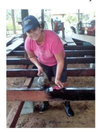
Ana Skelly paints the wood replaced when termites damaged the original. We replaced it with a hard wood that the termites don't like, then she treats it with a mixture of used motor oil and diesel.
